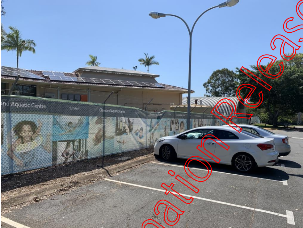
Figure 83: Public carpark where chlorine truck unloads
