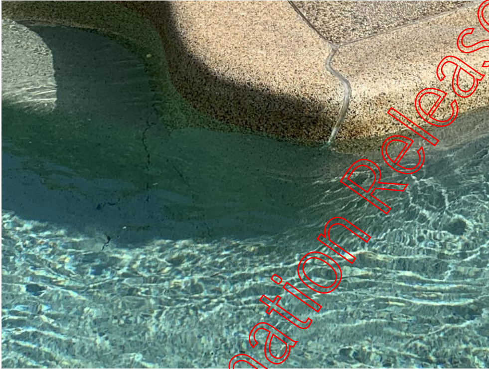
Figure 53: Cracked bench
