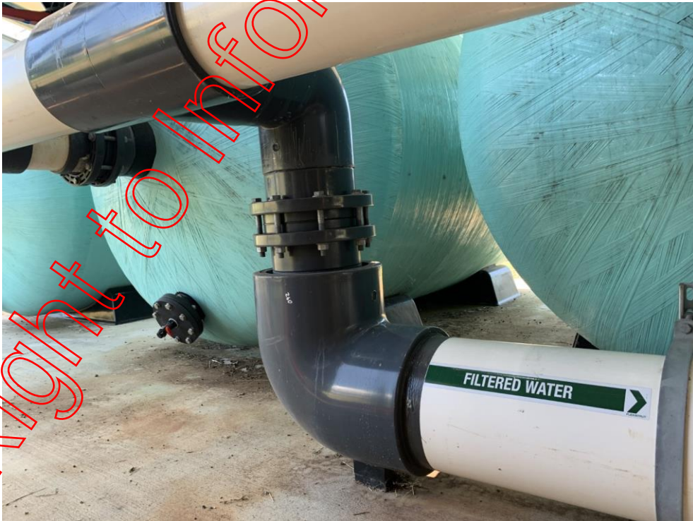
Figure 68: Late increase in pipe size
