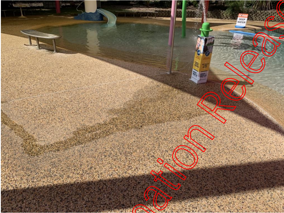
Figure 37: Water constantly leaking from cannon
