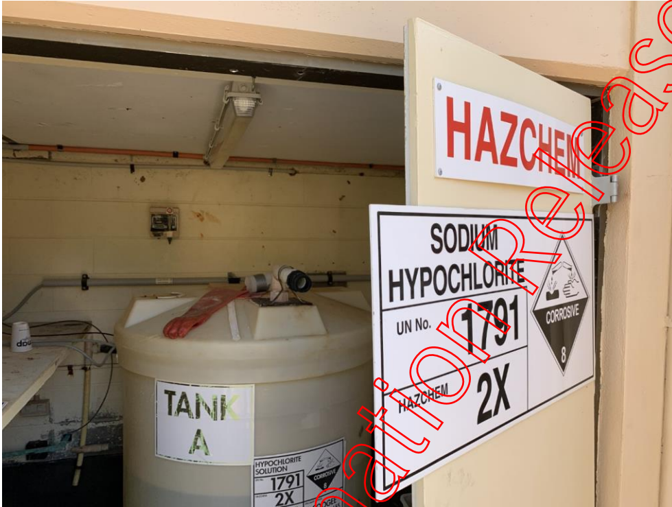
Figure 89: Poorly installed signage on broken door
