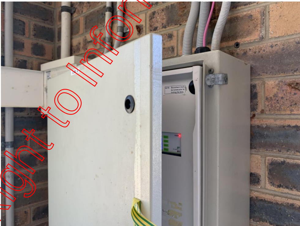
Figure 64: Conduit clip to hold door closed
