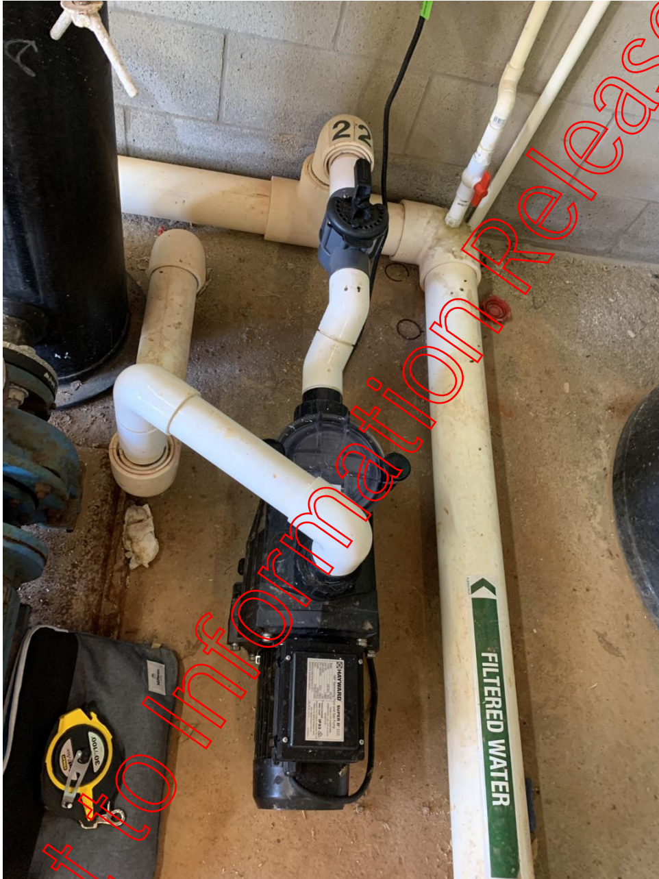
Figure 135: Disused boost pump, possibly for waterfall
