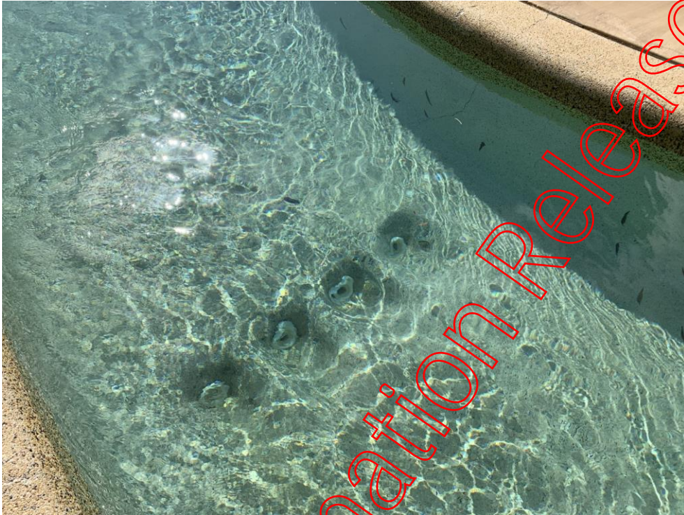
Figure 57: Jets in pool floor
