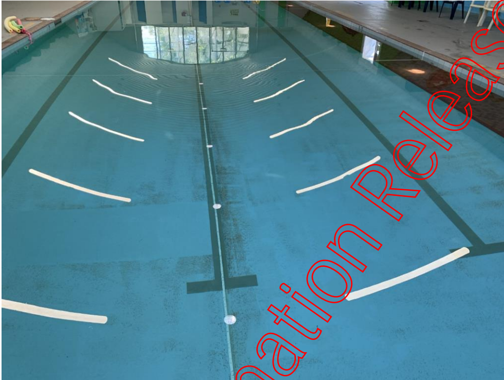
Figure 26: Wearing floor finishes
