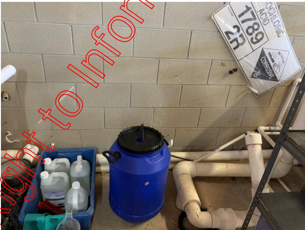
Figure 116: Poorly managed acid storage
