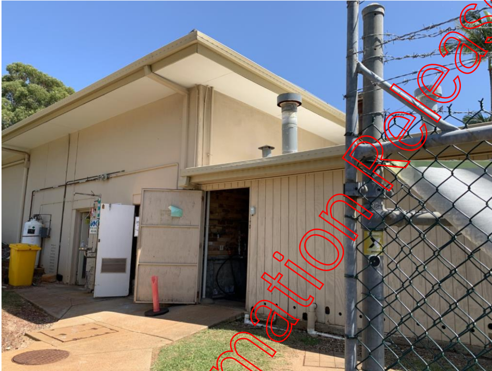
Figure 74 Eastern Equipment Room
