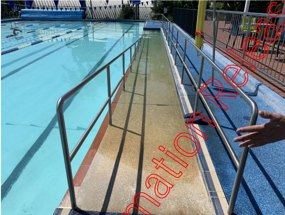
Figure 16: 25m Access Ramp
