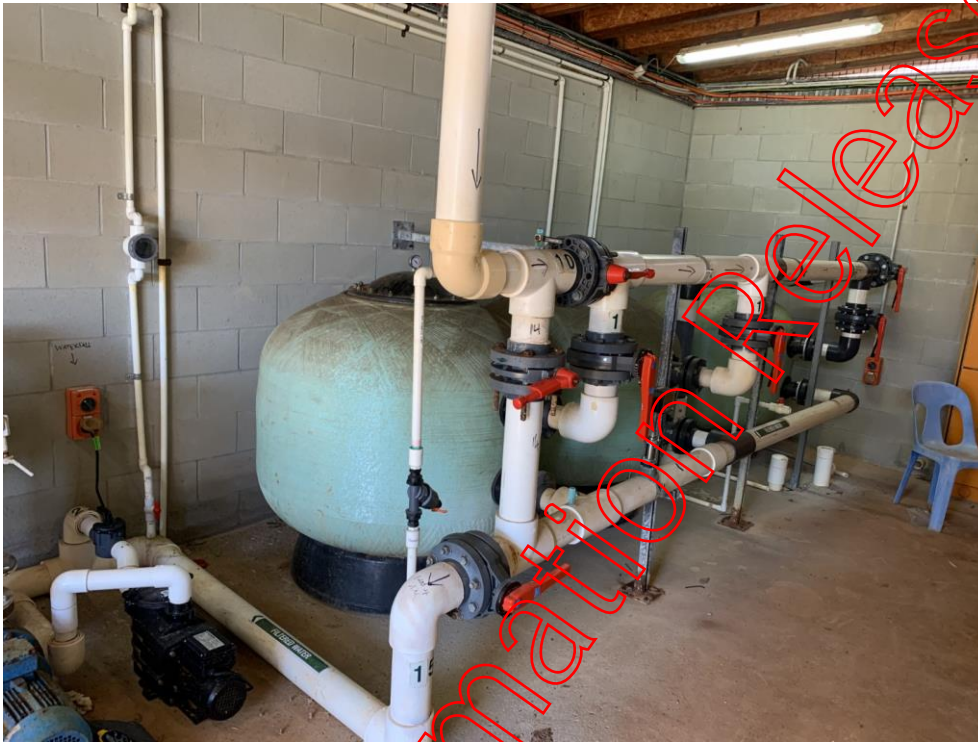
Figure 127: River Pool Filters
