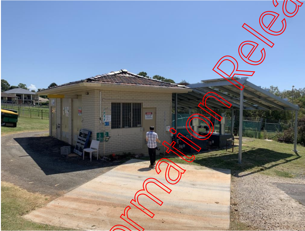
Figure 60: 50m Pool Equipment Room
