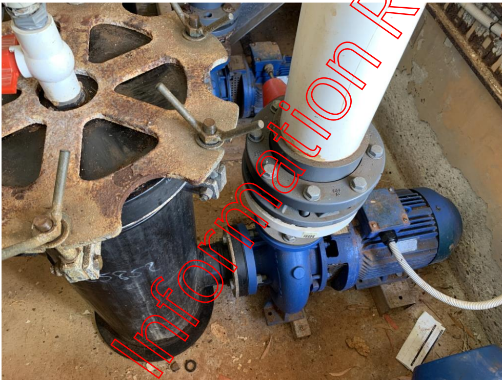
Figure 124: Filtration pump
